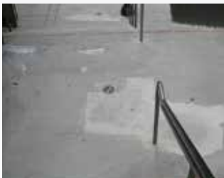
Resurface old, damaged concrete
