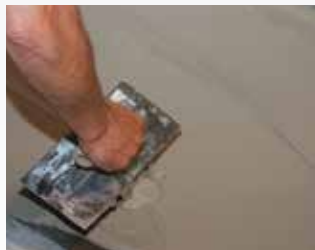
Apply using a squeegee or flat trowel up to 1/2 inch
